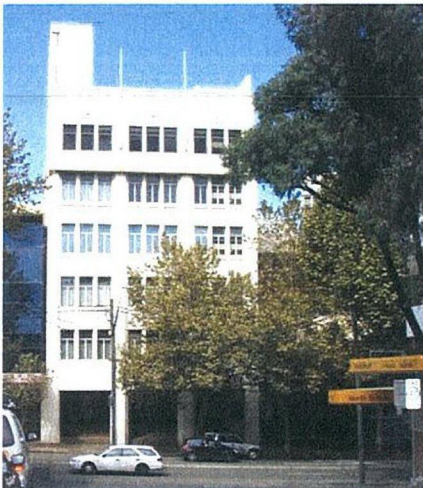
Figure 9: Existing site condition (No. 223) viewed from Doohat Avenue
