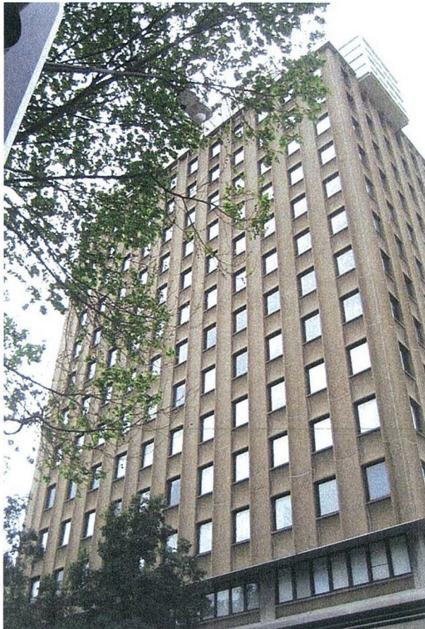
Figure 4: 229 Pacific Highway (approx 15 storeys)
